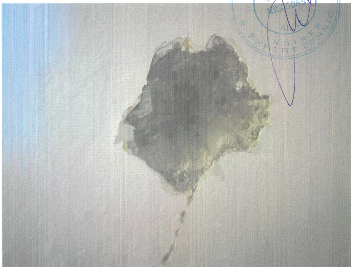
Identificare tip si diametru armatura in camp ( \Phi 8/30\text{cm} PC52)
